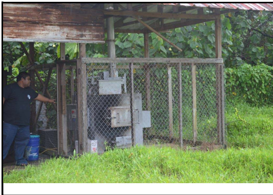
Photo 10: Incinerator used at Pohnpei State Hospital – wood used as a fuel source. (taken 7/04/2014 by Natalie Stella ref:DSC0101)
