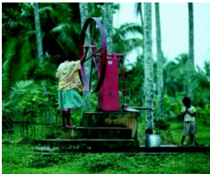
Village water supply, Kiriwina (Photo: Rocky Roe)
