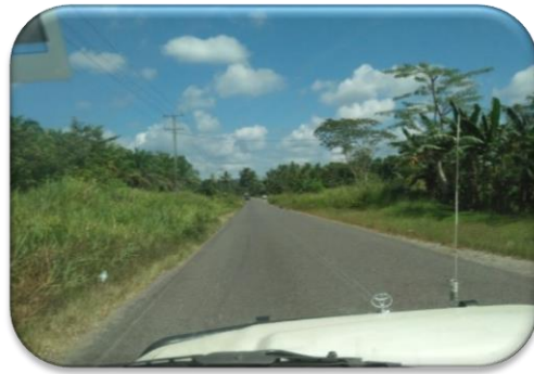
TRANSMISSION LINE SAGGED ALONG ROAD
