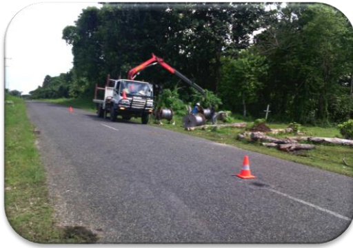
CRANE TRUCK ERECTING POLES
