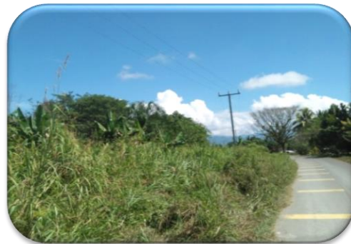
POLES SAGGED AND ERECTED ANGENABO
