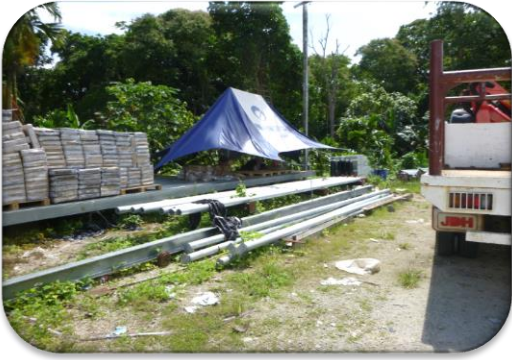
LAYDOWN AREA KOKOPAU
