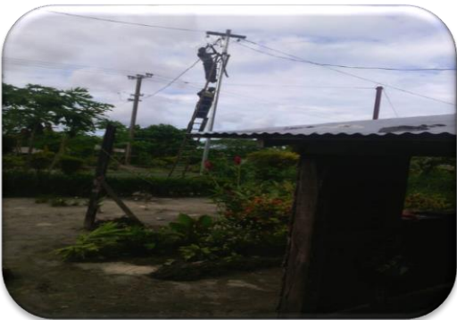
LINESMAN CONNECTING HV LINES
