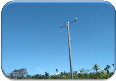
POLE ERECTION AT POPONDETTA
