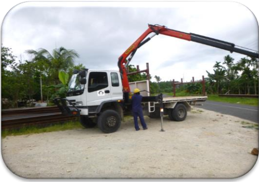
CRANE TRUCK ERECTING POLES
