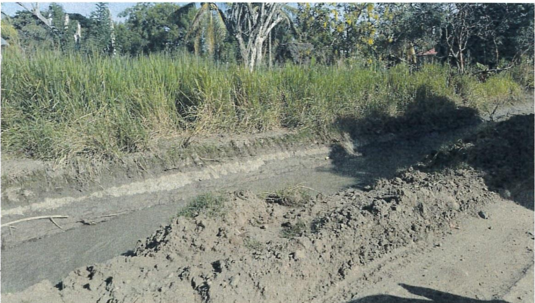
Photo 6 (Zone 1) showing a stream flowing down temporary drains by the Highway. This is possibly due to a recent shift in a tributary, leading to part of the tributary now following the Highway's course
