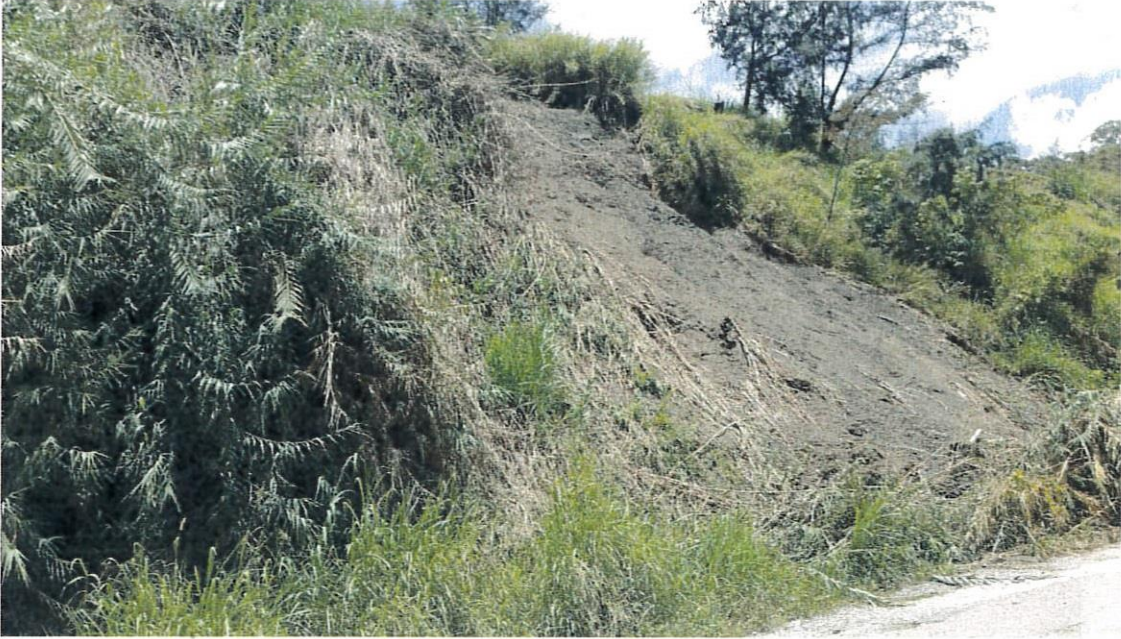
Photo 13 showing one of many recent minor landslides, this one in Zone 3
