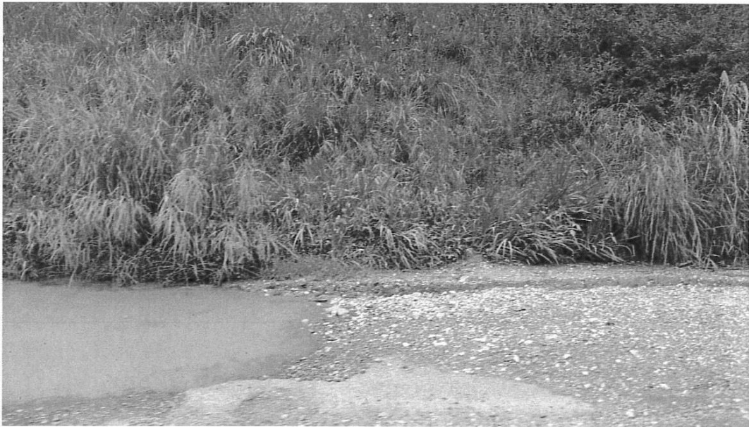
Photo 12 showing water lying on the road surface in Zone 3 – this is evidence that the water table lies close to or above the road surface
