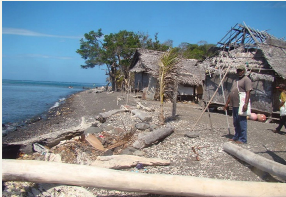
Coastal erosion at Kavailao Bay, Karkar Island.
