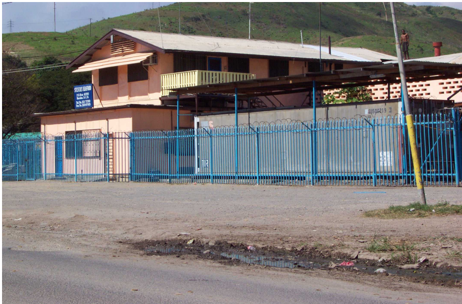
Photo 17: Typical Industrial Building in Newtown
