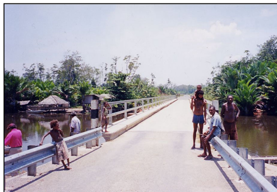
Section of the Bereina-Malalaua Road
