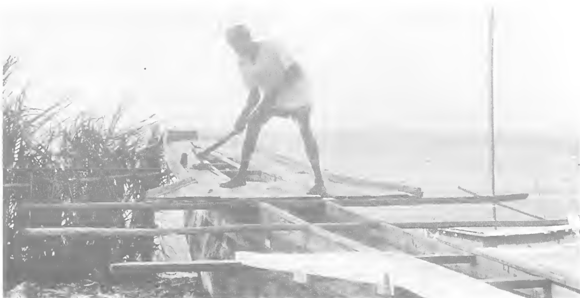
FIG. 56. Adding a platform deck and planked sides to a canoe hull using adze fitted with a metal blade, Kadawa village, SW coast.
