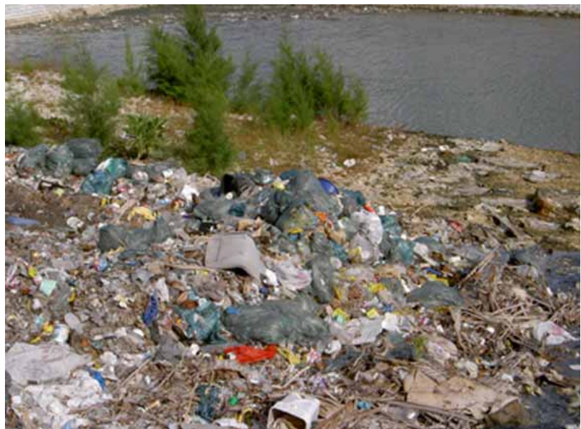
Figure 18: Filled area of Nanikai Landfill in October 2004. Note water in the bottom right corner, indicating that filled area is less than the access roadway in the centre of the picture.
