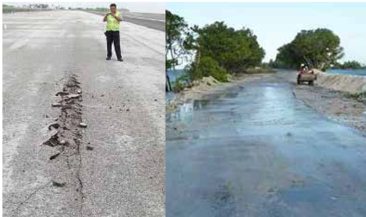
Photo 16: Major Erosion at Majuro airport and catchment, caused by Upwelling during the February 2011 King Tide
