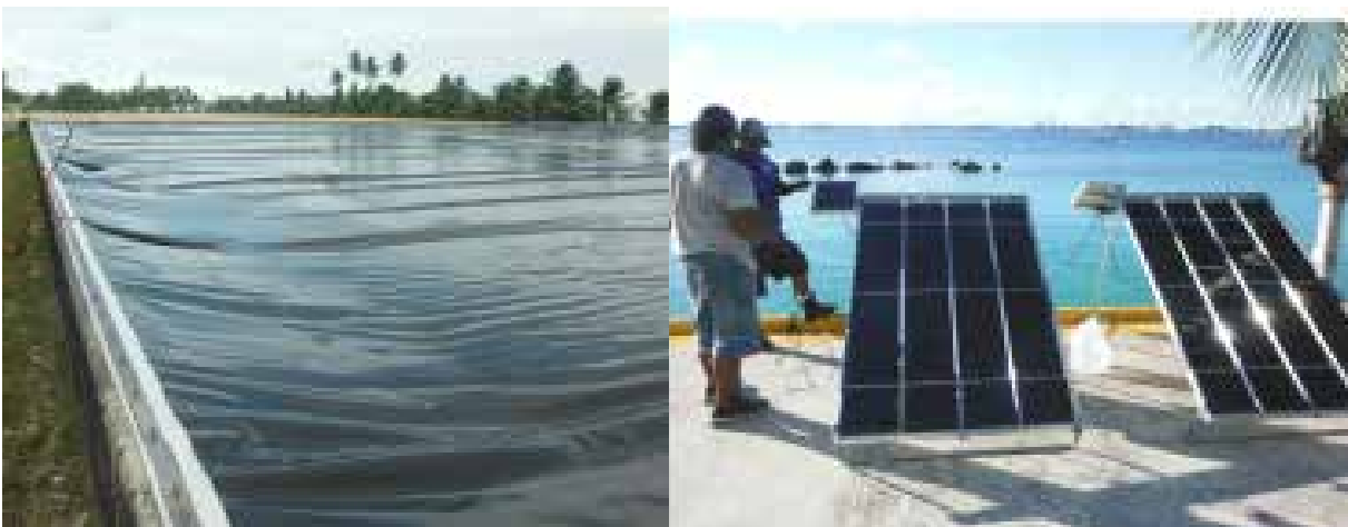
Photo 18: Reservoir in Majuro
