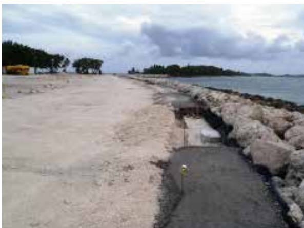
Photo 8: Construction of Runway Safety Area (RSA) Barrier Wall
