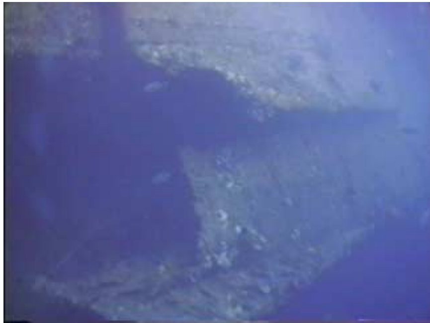
Photo KS13-4 Hull damage from triple torpedo mount explosion.
