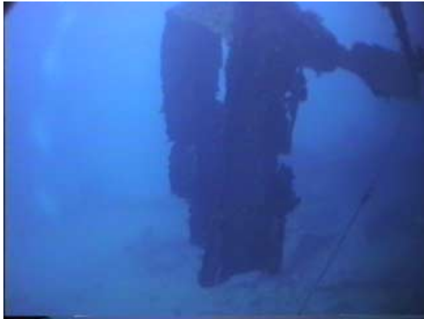
Photo KS13-7 Hanging hull section from damage site. Section is attached to anti-submarine cable and extends almost to the sand.
