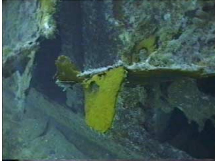
Photo KS4-8 Starboard side metal sheeting at engine room with sections pulled upwards. Rust on edges indicates recent movement
