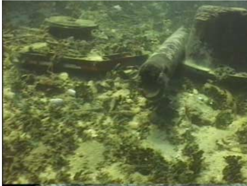
Photo KS8-4 New Ebeye Dock debris at old Japanese floatplane site. Debris is primarily large rubber fenders that have been torn off the dock face.
