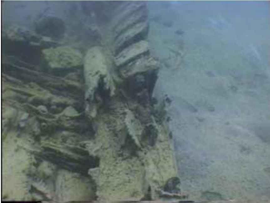
Photo WT7-2. The bow of the Central Vessel, with decayed bow spirit and residual concrete repairs between the frames on the port side obviously evident.
