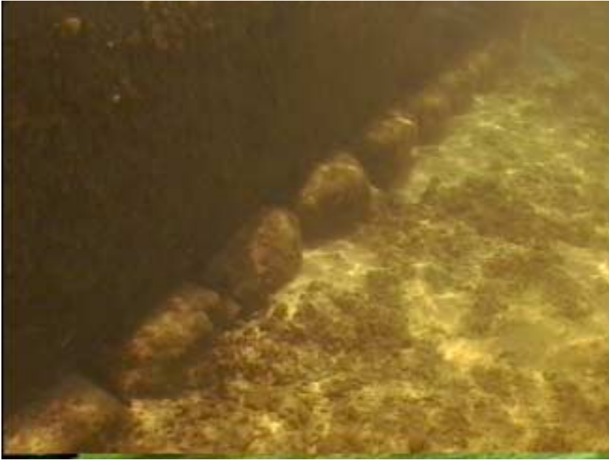
Photo WT4-4. Cement bags used as the Seaplane Ramp wall foundation.
