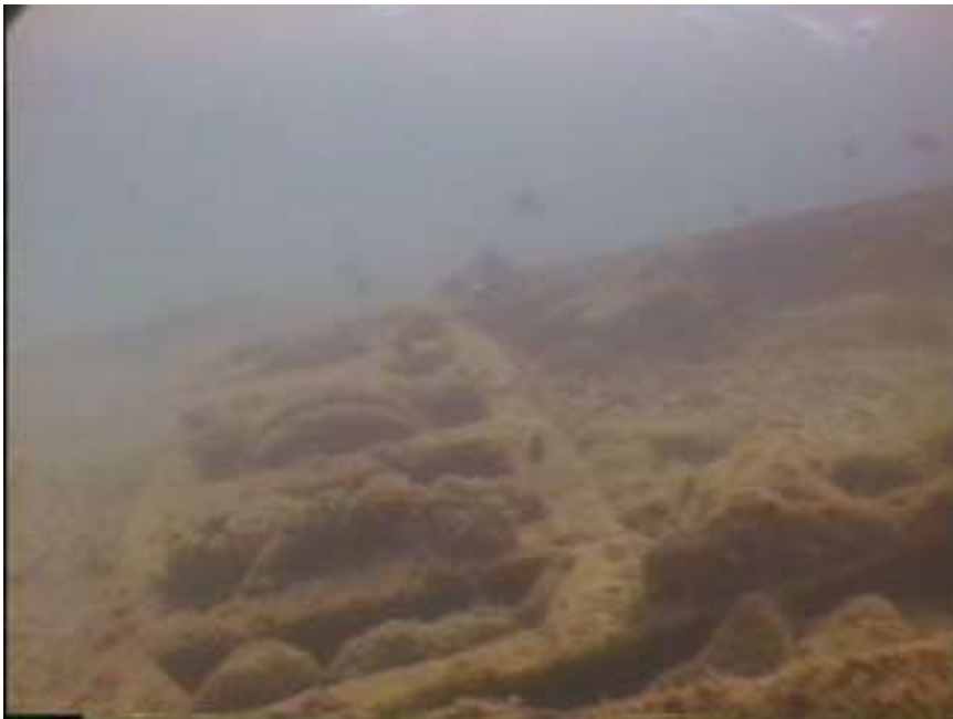
Photo WT6-3. Top of Crane section underwater off end of Main Service Dock.
