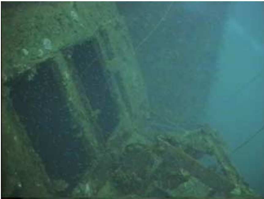
Photo WT12-13. Open engine room skylights.
