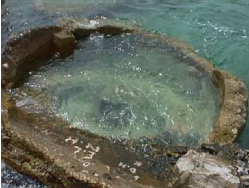
Photo WT6-4. Anti-Aircraft Site blown into water from bomb damage at the end of the Main Service Dock.
