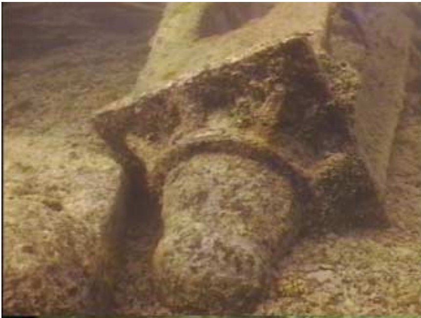
Photo WT6-5. Ships service tie up bollards at the end of the Main Service Dock.
