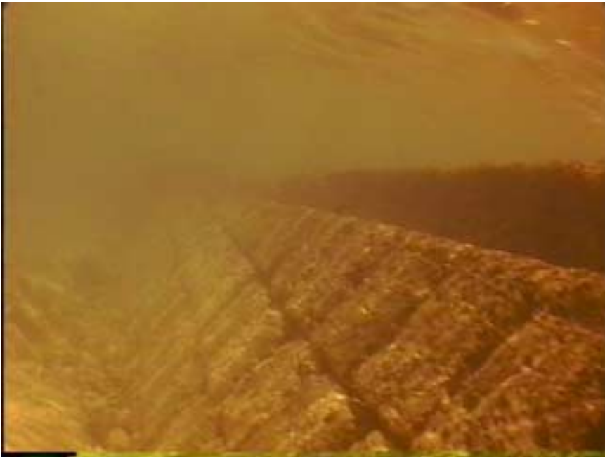
Photo WT4-5. Formed blocks laid for walls of the Seaplane Ramp.
