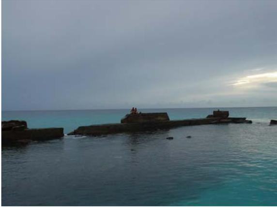
**Figure 11. Outer wall of pier, Taroa. Note the extensive deterioration of sections**
