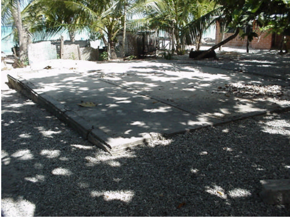
Photo 2 Warehouse foundation at Jaluit Company Trade Station
