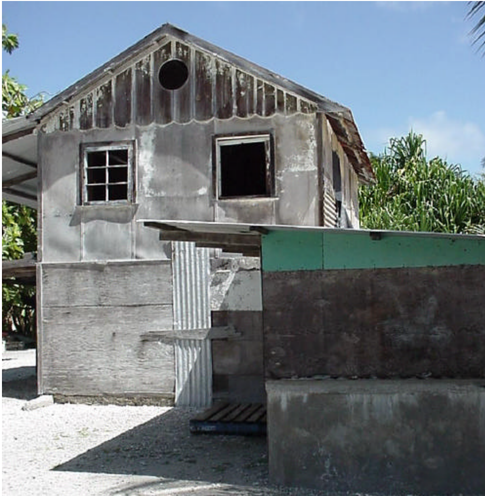
Photo 4 Japanese house foundation (used with present house).
