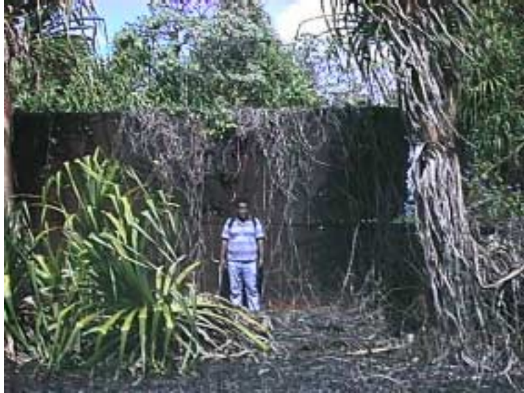
Figure 1. Interior walls of Tank One.
