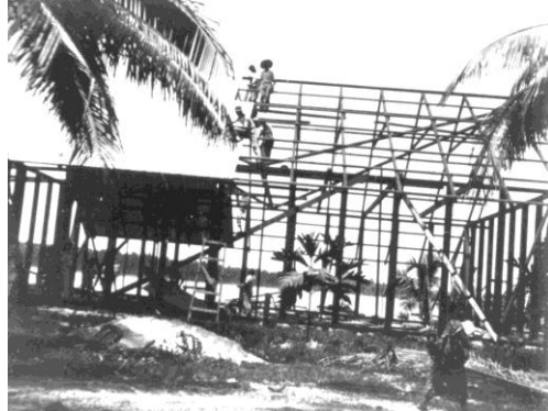
Photo 72: Construction of Old Copra Warehouse.
