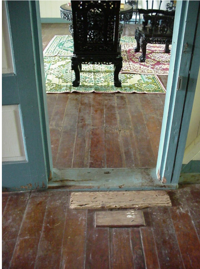
Photo 28: Wood Damage on Floor in Southern Bedroom.
