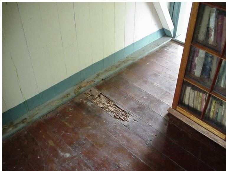
Photo 28: Wood Damage on Floor in Southern Bedroom.
