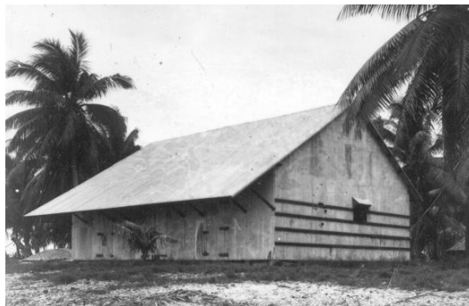
Photo 73: Old Copra Warehouse.
