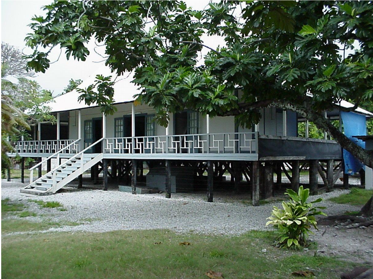
Photo 10: Joachim deBrum House, taken from Southwest corner
