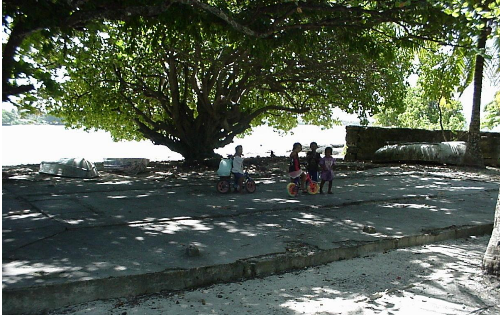
Photo 64: Community Hall foundation.
