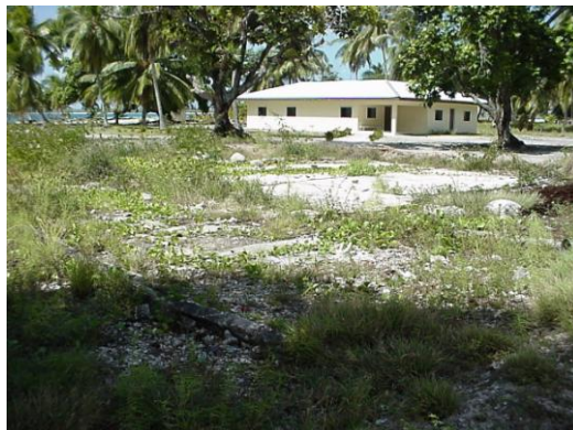
Photo 74: Concrete Slabs of Old Copra Warehouse.
