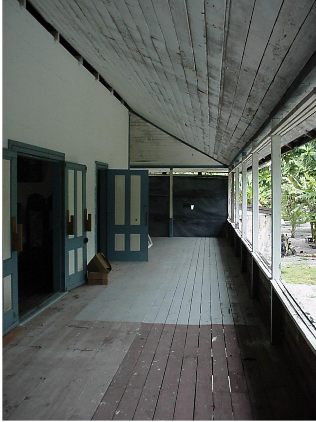
Photo 12: East Veranda of deBrum House, looking north.
