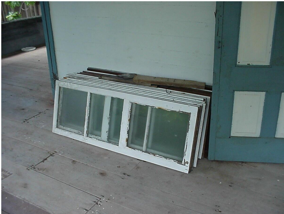
Photo 15: Sliding glass plates removed for construction.
