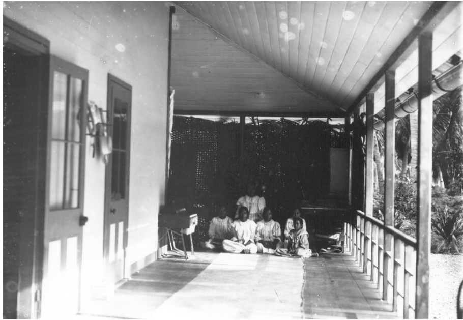
Photo 13: East Veranda of deBrum house, circa 1900.
