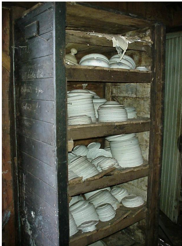
Photo 35: Damaged shelving with china, inside storage shed.
