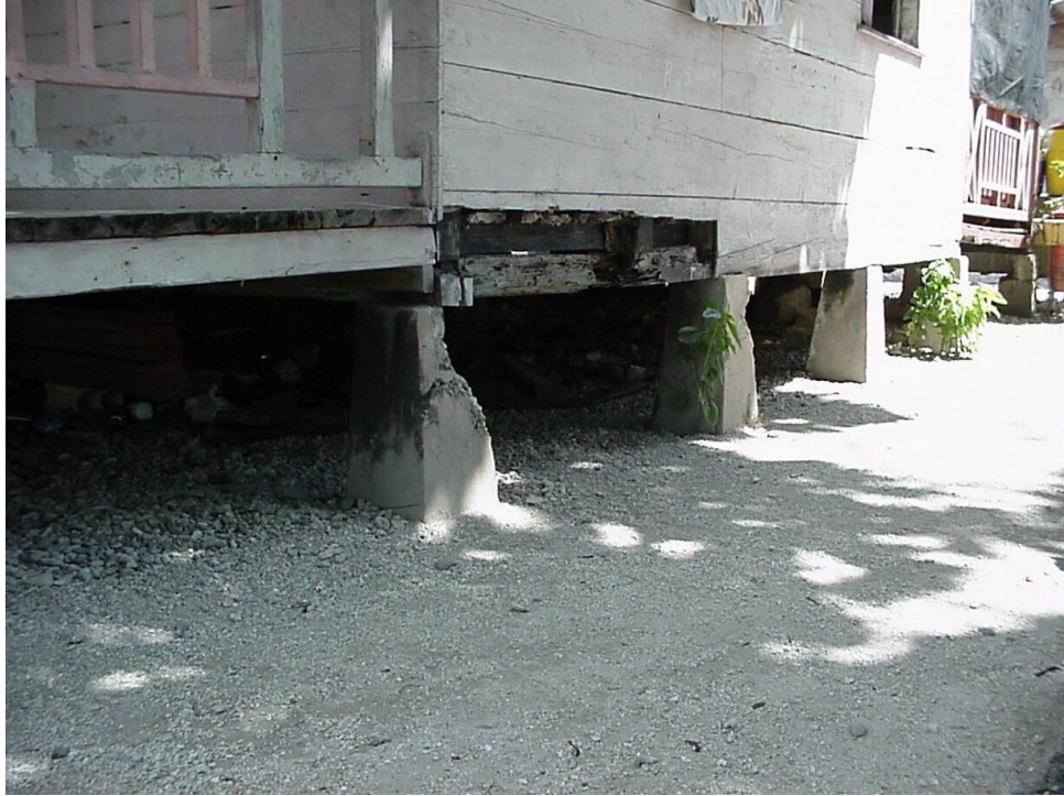
Photo 62 Closeup of pillars from Elise deBrum Hahn house.
