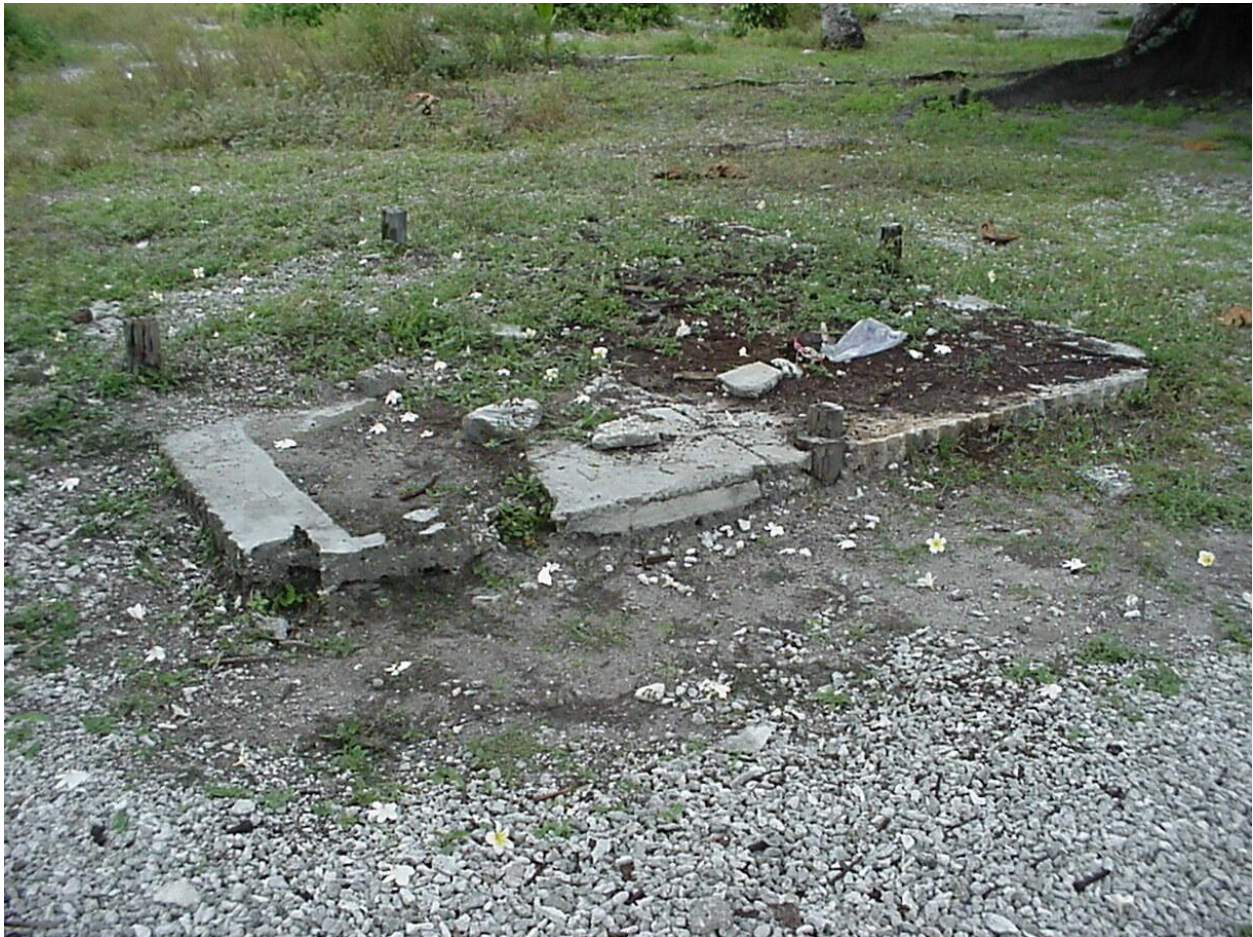
Photo 36: Original Darkroom foundation.
