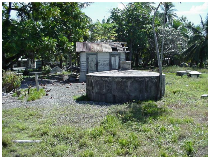
Photo 50: Water catchment and Pump house of Likomju deBrum
