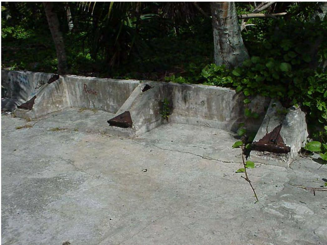
Photo 81 Hangar Wall and Roof foundation.
