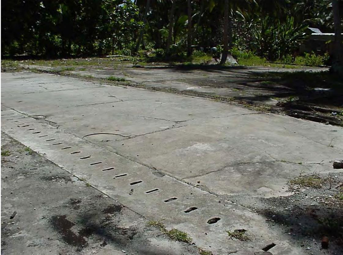
Photo 57 Hangar foundation and drainage.
