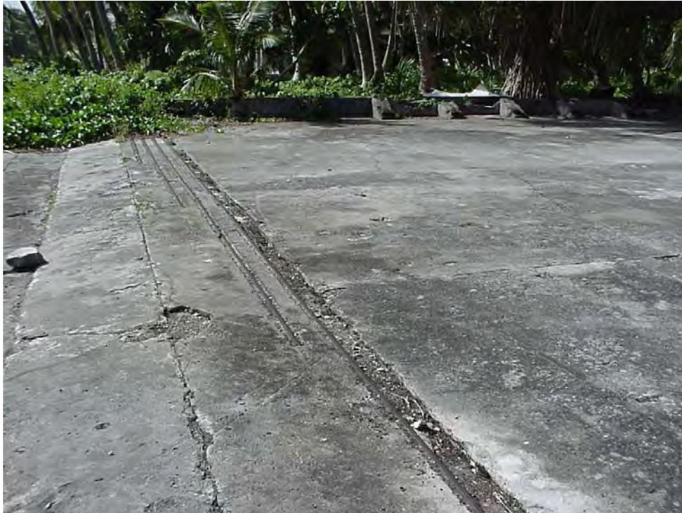
Photo 80 Hangar (rails for sliding doors).
