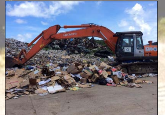
EXCAVATOR SORTING AREA AND LANDFILLING WASTE
