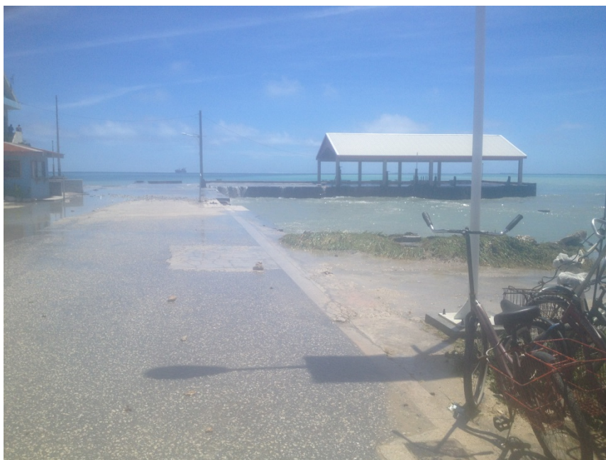
Figure 7.8 Inundation of the area near the harbour due to westerly waves from the lagoon.
