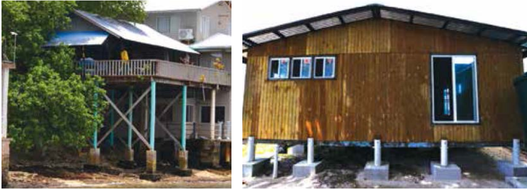
Figure 10.1 Elevated houses in Majuro to prevent damage from waves and flooding (Hess et al., 2015).
