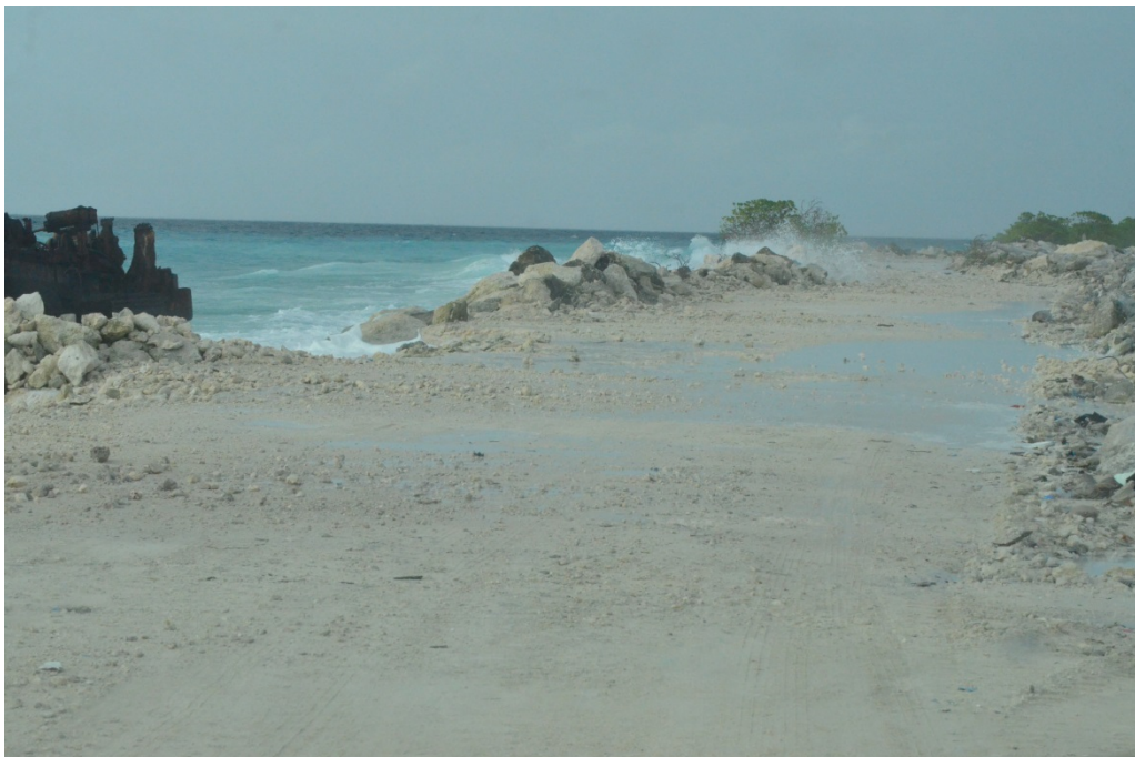
Figure 7.16 Picture of the causeway after a mild storm events on the 19th of August 2016. Debris was brought by the waves on the causeway.
