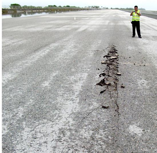
Figure 20. Hydrostatic pressure damage to the Majuro airport catchment, caused by upwelling during the February 2011 king tide (photo courtesy RMIPA).
