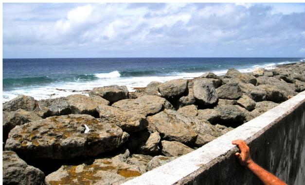
Figure 8. Ocean-side concrete wall and armor rock.
