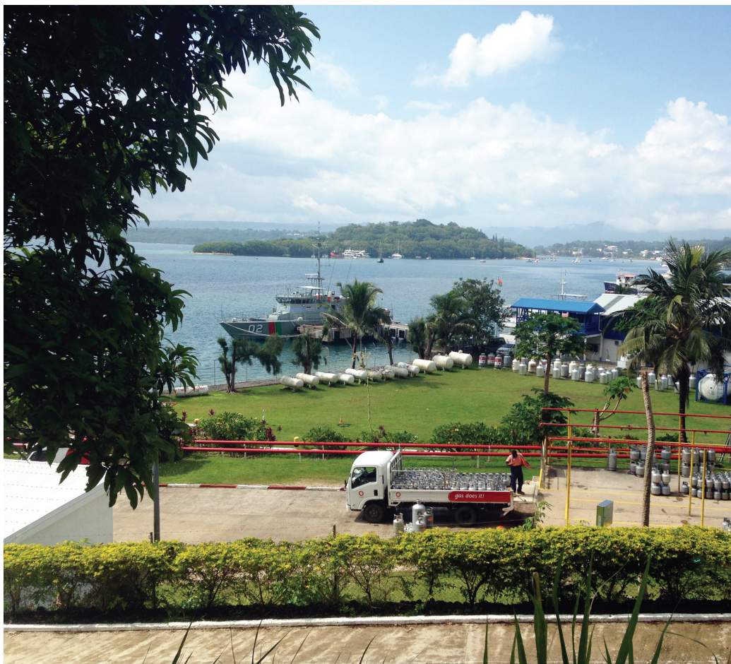
Origin LPG depot, Port Vila Photo: H. Wade
