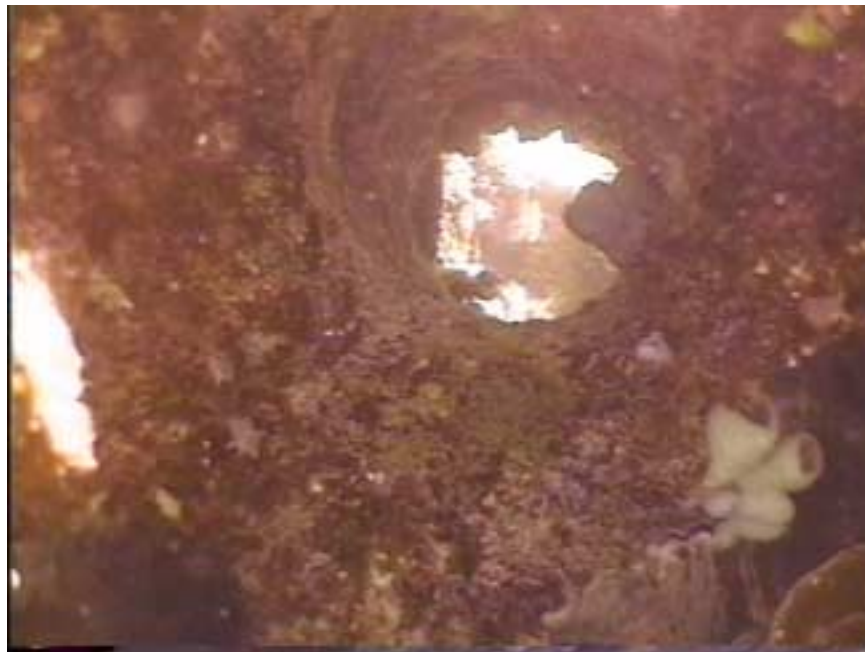
Photo MS4-6 Hole through concrete "Dead-man" where telephone pole was originally placed in concrete.
