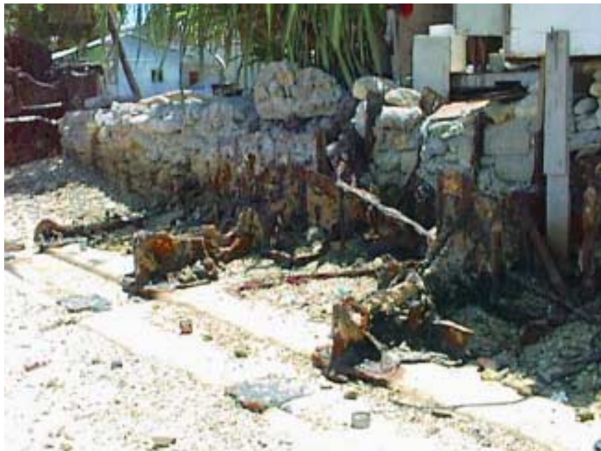
MS6-1 Shore-side attachment point on the US dock at Rita. A section of barge was set in concrete on the hard reef at the shoreline.
