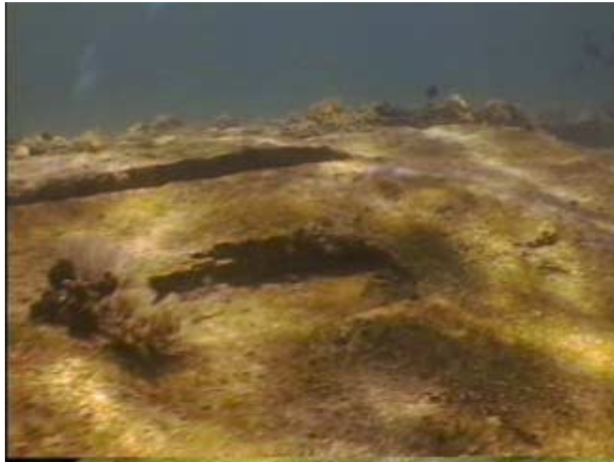
Photo MS4-7 Concrete pour for top of wharf now lying on the bottom
