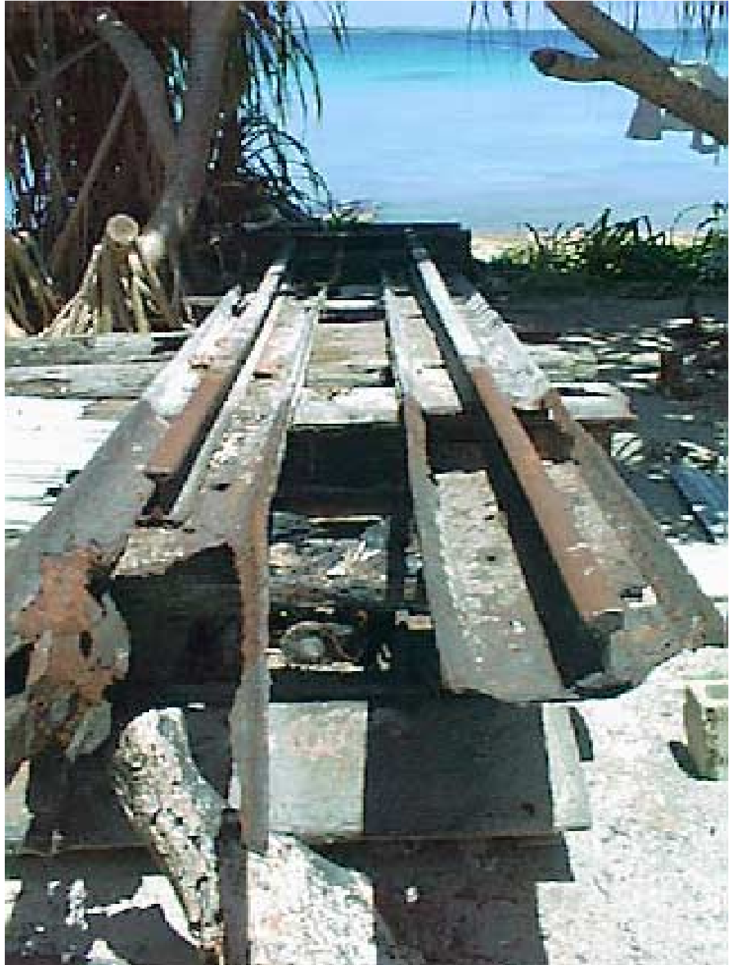
Photo MS7-1 Shore side end of Marine Railway, north track section. Note the sheet pile and heavy timber foundation.
