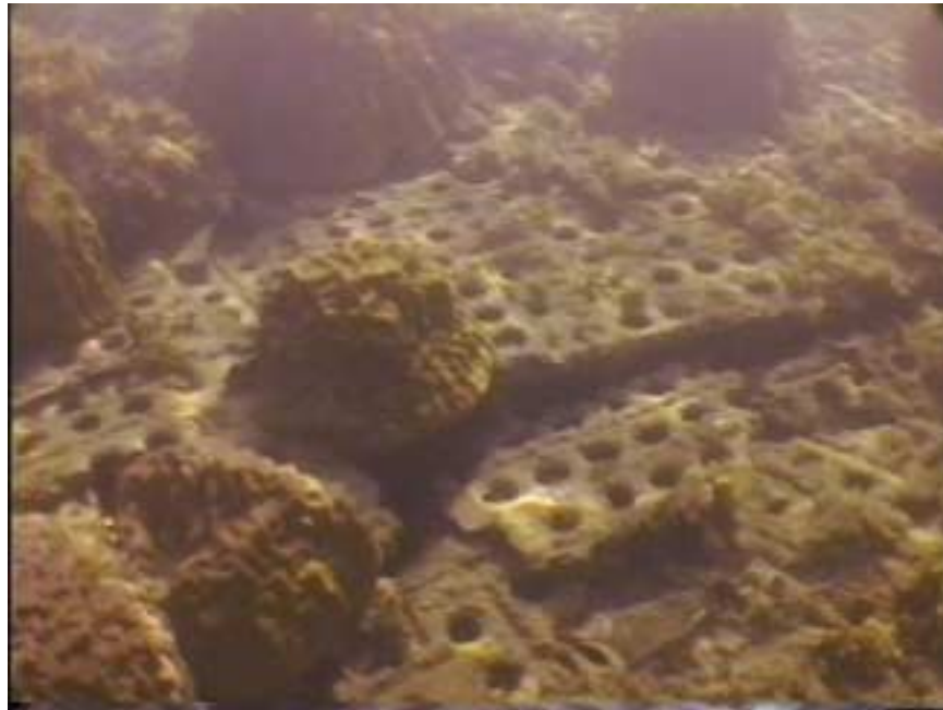
Photo MS7-4 Majuro Seaplane Ramp with Marston matting.
