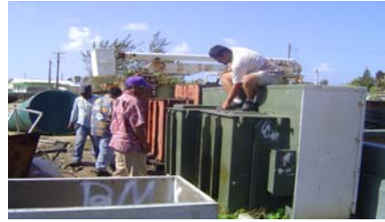
Testing of 20 + transformers in Ebeye
