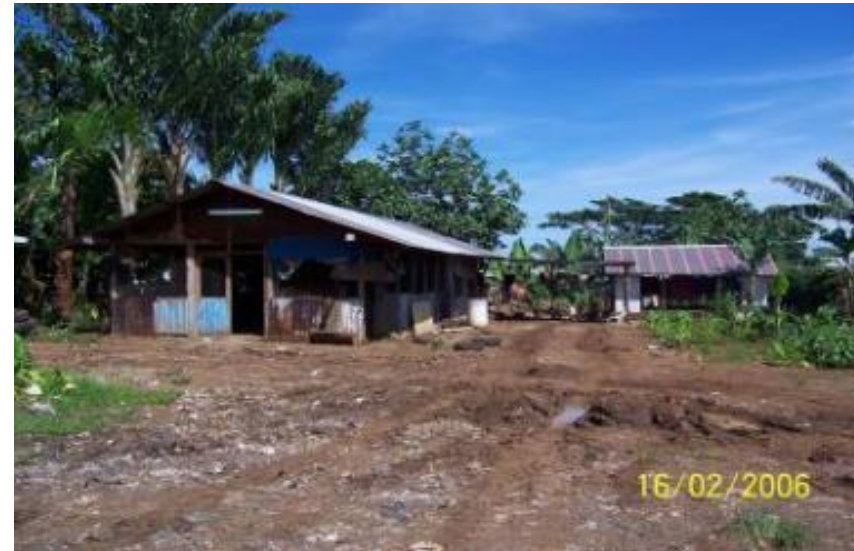
Plate 1: Old Vaitele SLC Subdivision – poor access and drainage
