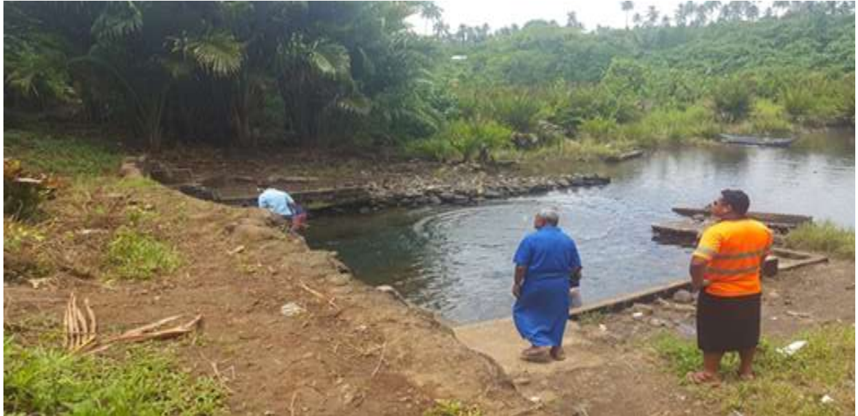
Coastal spring (Puna Lafa) next to wetland in Salani - potential contamination from nearby households with latrines located above the pool.
