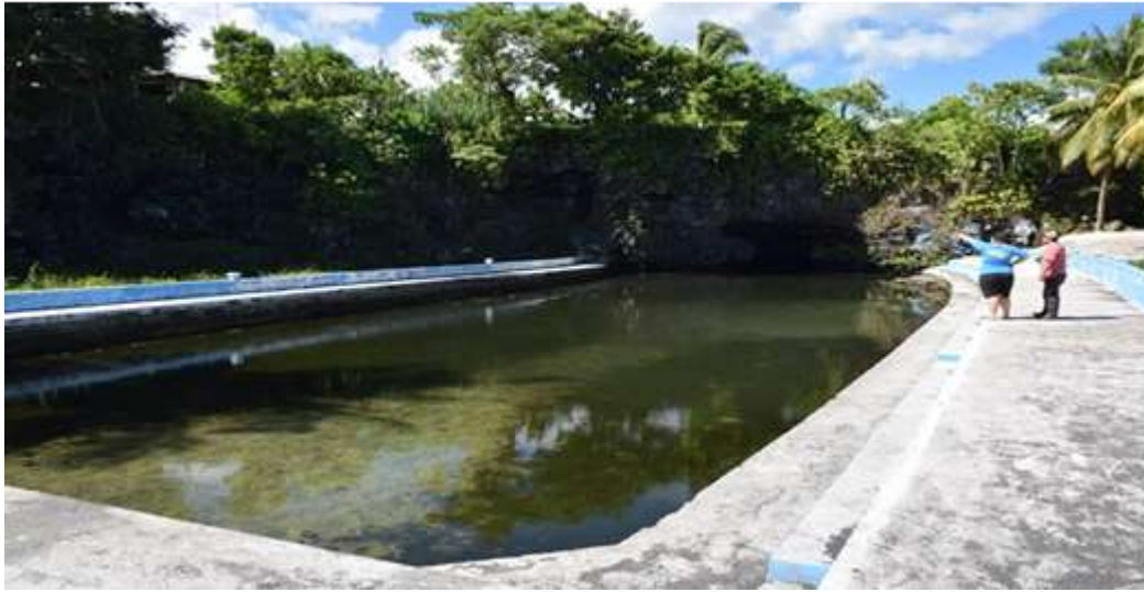
Taga Village pool So'otuna upgraded under the PPCR-ECR small project
