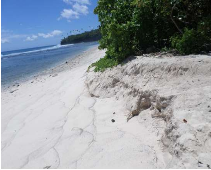
Evidence sand mining practice Foailalo old village near the coast.
