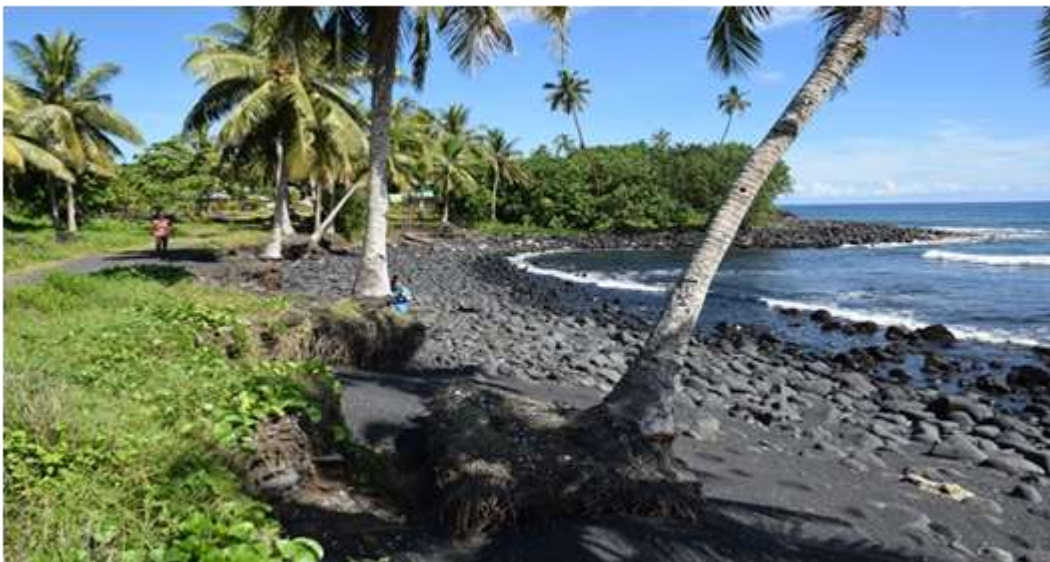
Taga old Village on the coast highly eroded almost reaching road.
