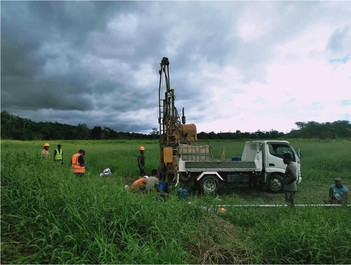
Plate 11. Drilling of BH4.
