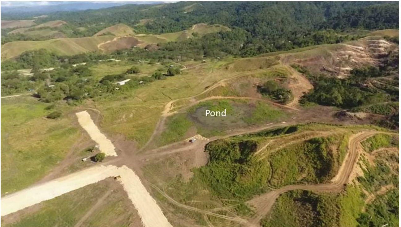
Plate 5. View south towards Poha and LD, note formed accessway
