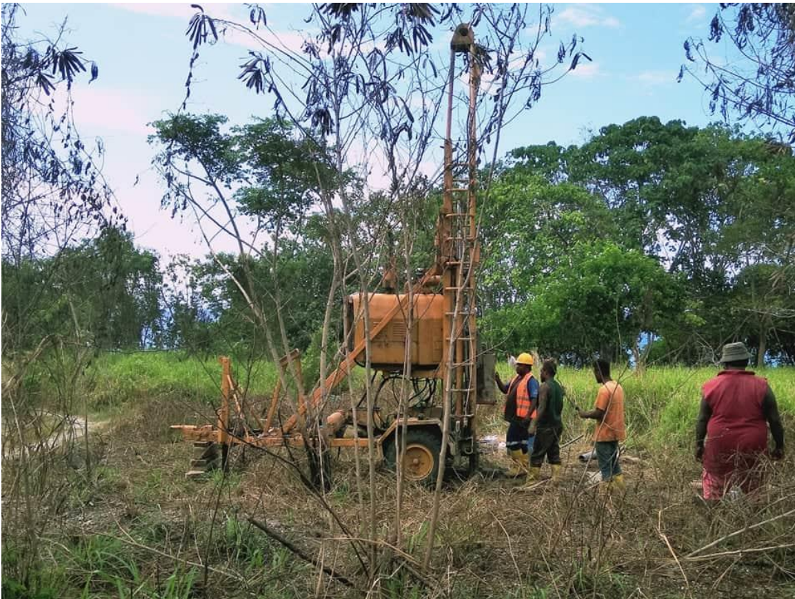
Plate 10. Drilling of BH1 near the coat.
