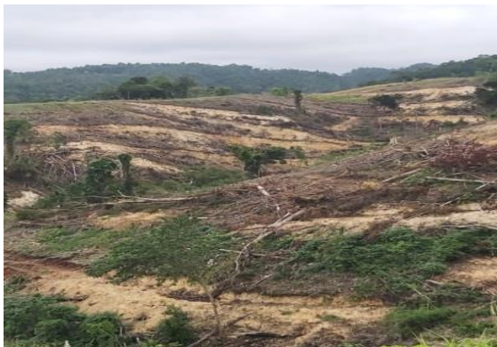
Hills clearing and backfilling
