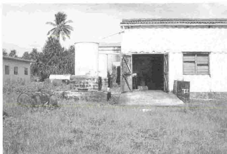
Back door of Funafuti Power Station. Oily wastes are simply hosed out the door, and drain away into the groundwater below. Managing oil waste is one of Tuvalu's most urgent pollution issues. (photo: Alefaio Semese)
