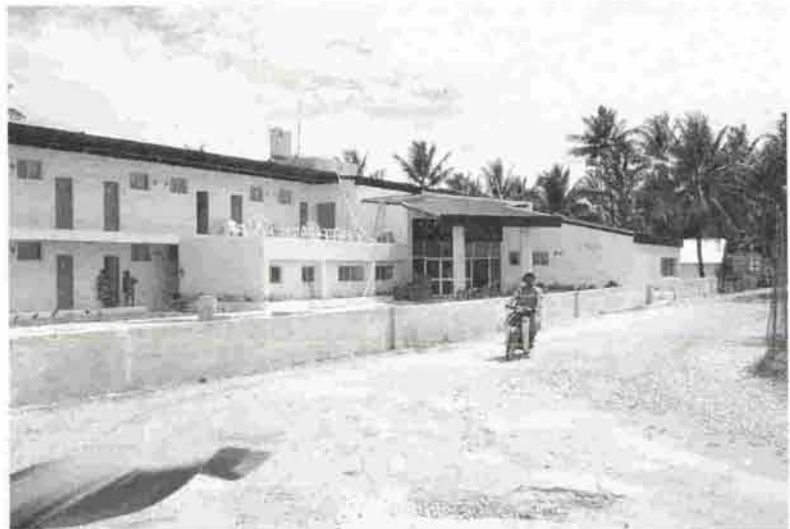
Vaiaku Lagi Hotel. Donor-sponsored development such as this will provide a great economic boost to Tuvalu. However, such developments should be subject to Environmental Impact Assessment (EIA) to ensure they meet agreed building and environmental standards. (photo: Alefaio Semese)
