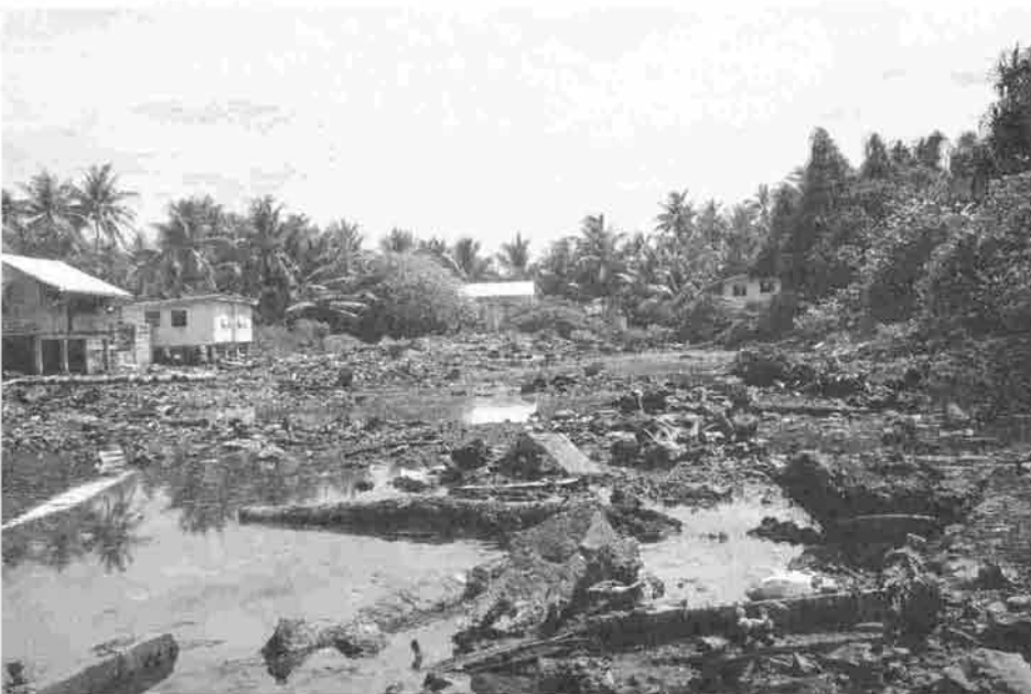
With rapid population growth land is in short supply. These people are having to build over one of Funafuti's borrow pits. The pit is also used for rubbish and receives animal waste. (photo: Alefaio Semese)
