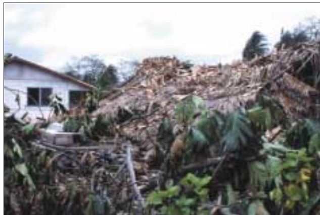
Damages caused by a storm on Vaitupu Island (photo: McQuarrie)
