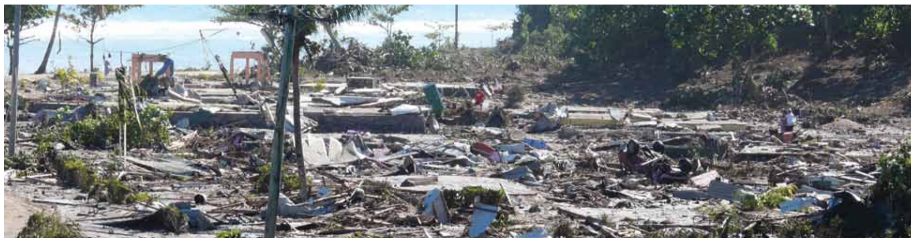
Figure 2. Aftermath of the 2009 Tsunami at Lalomanu, Aleipata, Samoa. Photo: J. AhKau and M. Leavasa.
