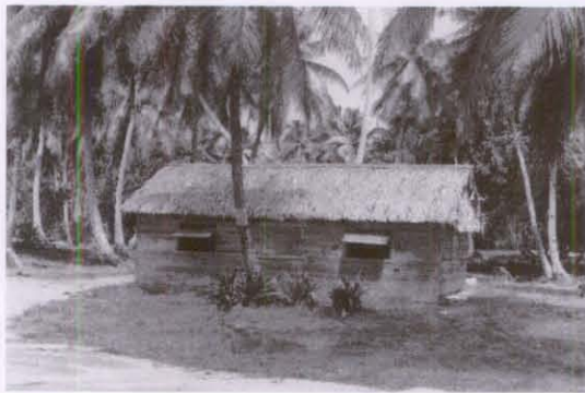
Fig. 48. School building in 1961.
