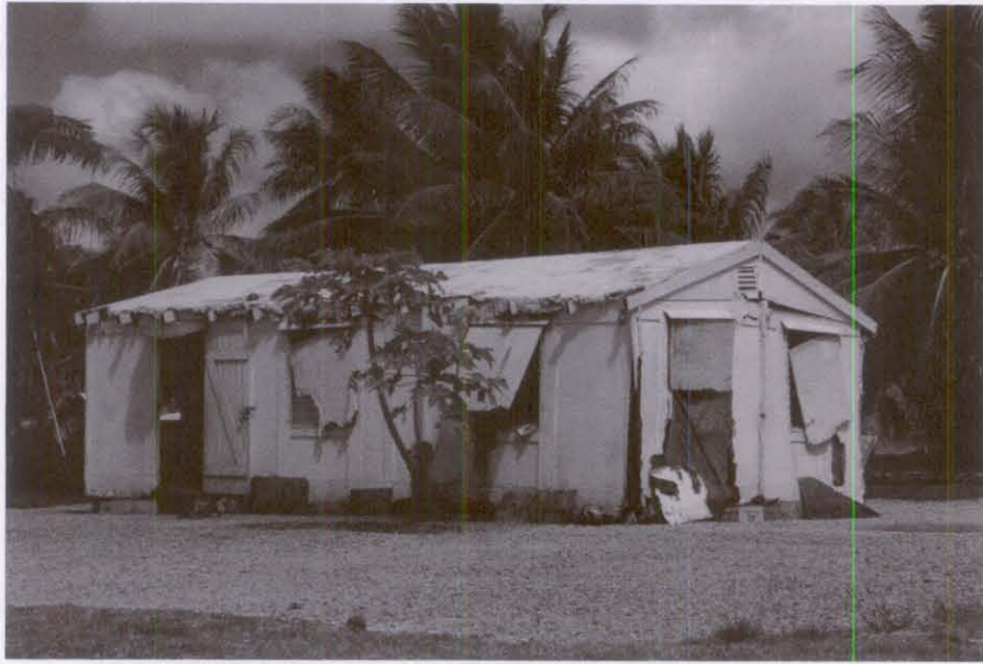
Fig. 42. House on Wotho Island, built by FEMA in 1992.
