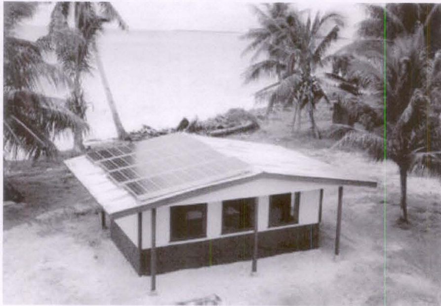
Fig. 55. Photovoltaic-powered freezer unit on Wotho Island, 1991.
