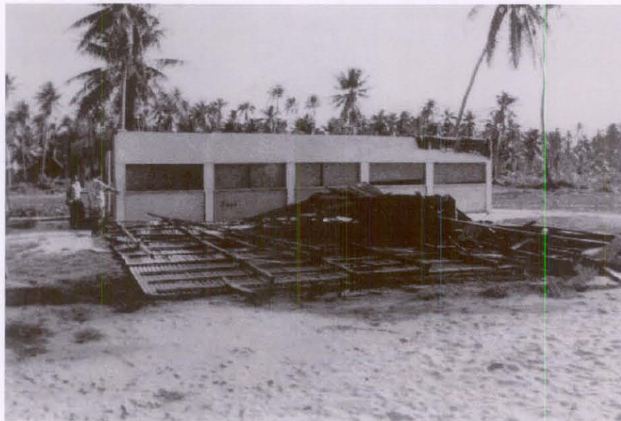
Fig. 41. Damaged school building, typhoon Pamela, 1982.
