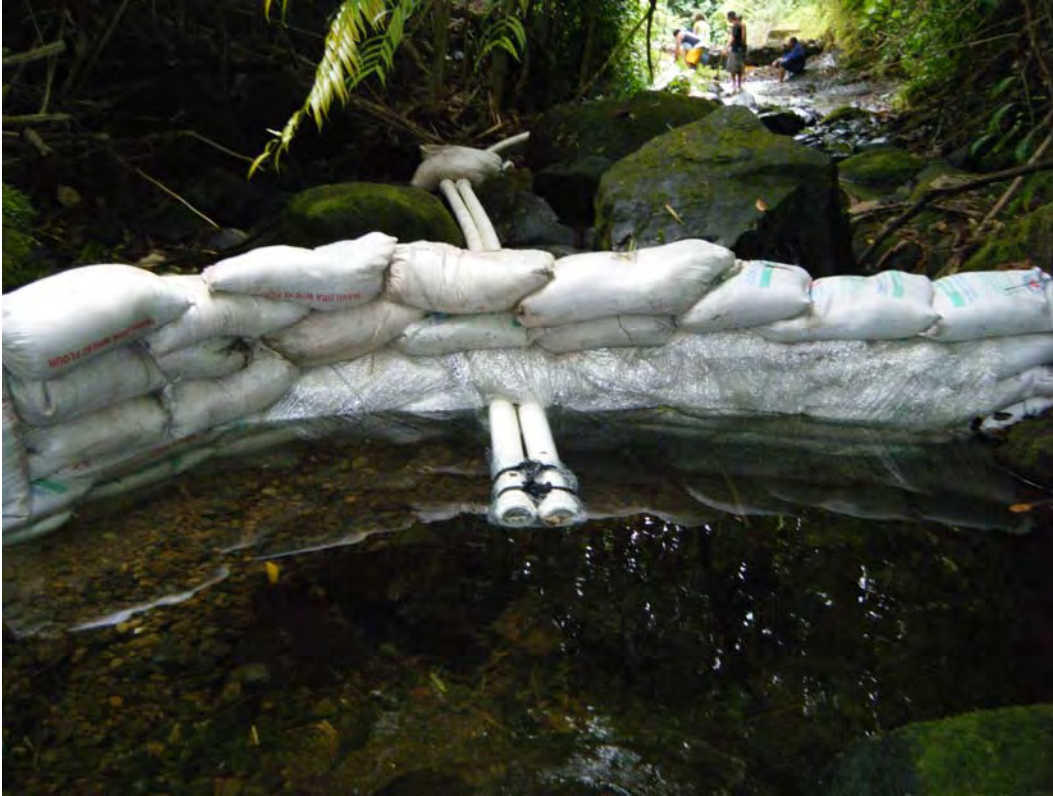
Figure 4: Sandbag dams to collect alternative water sources at Avatiu intake constructed during November 2009 drought (Obtained from MOIP, GOCI)
