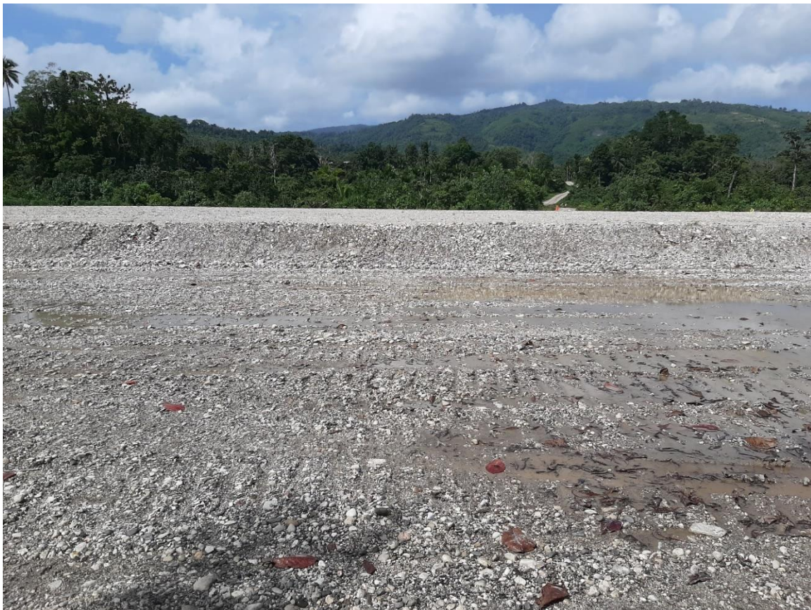
Fig 1, Backfill area proposed for the development
