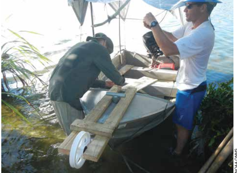
Figure 29: Building the tow pulley on the bow of the skiff.
