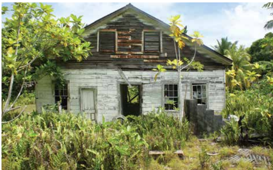
Figure 147: Back of Jennings residence and concrete steps.
