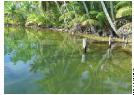
Figure 91: Three wooden pilings extending out from the southern shore of the lagoon, one submerged.
