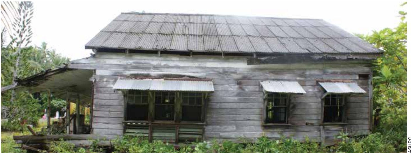
Figure 148: Showing southeast side of Jennings residence in Etena.
