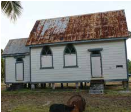
Figure 176: South side of church at Taulaga.
