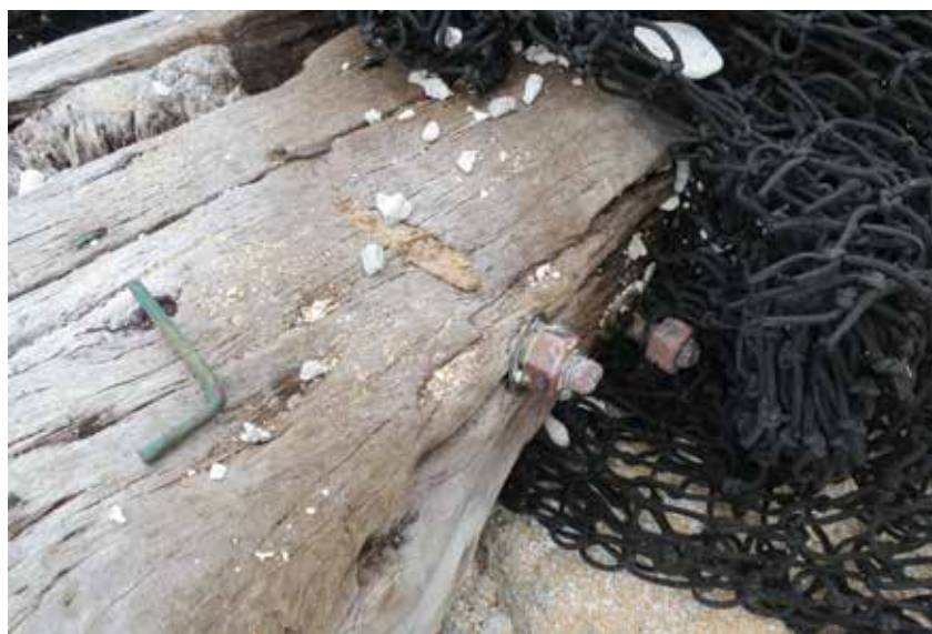
Figure 121: Ends of the threaded through-bolt fasteners.
