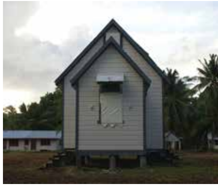
Figure 175: West side of church at Taulaga.
