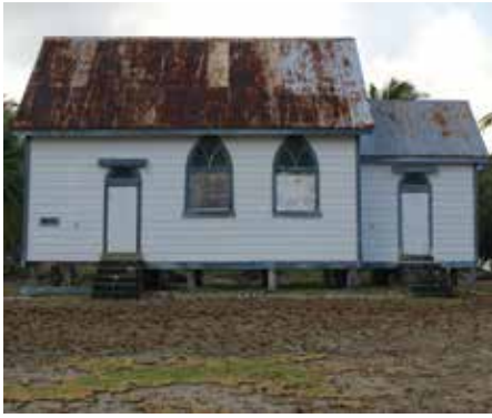
Figure 174: North side of church at Taulaga 2013.
