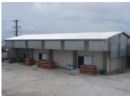
Image 21. KFC Cold Storage Facility
