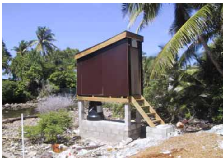
Figure 4A: Alternative human waste management system (individual composting toilet system)
