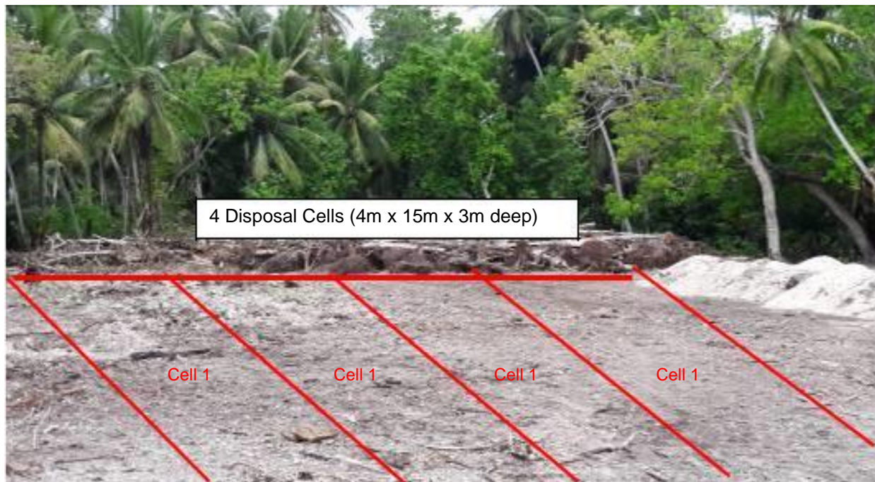
Marking of smaller cells on the cleared area
