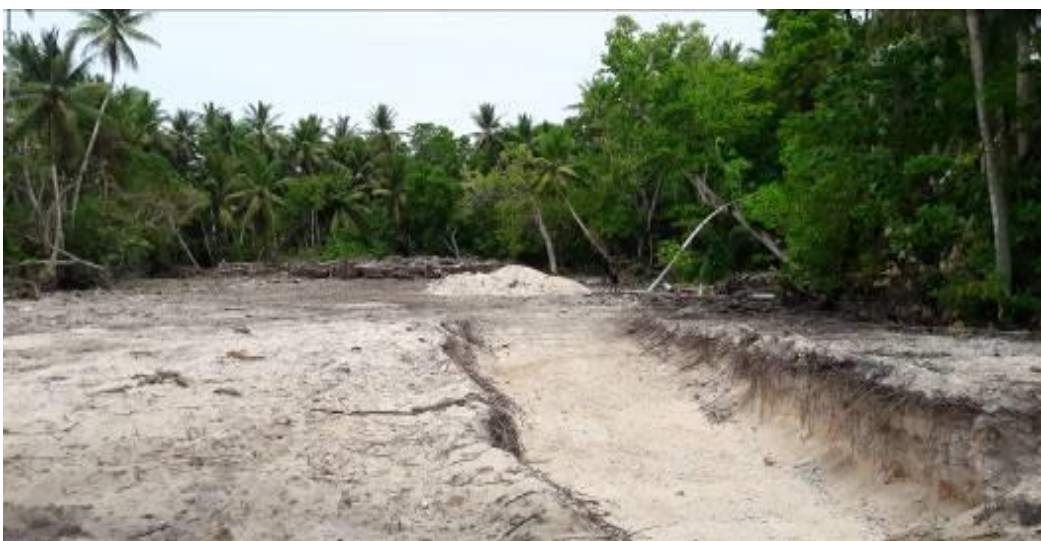
Photo 27: Created open ditch for Waste Disposal at Manumea
