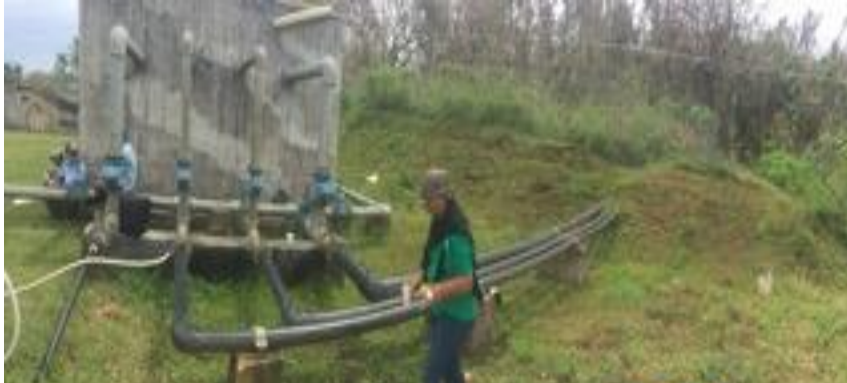
Figure 3 TWB reservoir field. Assistant geologist 'Amelia Sili is standing in front of the individual pipeline from different springs.
