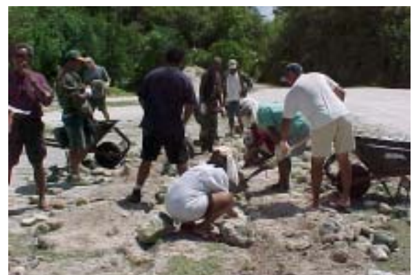
Construction of the flowerbed stonewall at Southern Community Health Center, Peleliu
