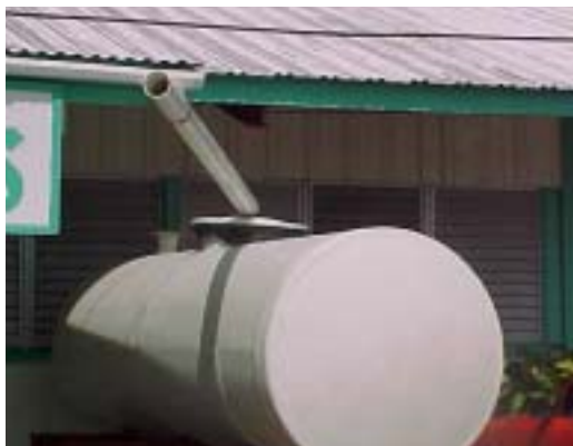
Household Water Catchment Tank
