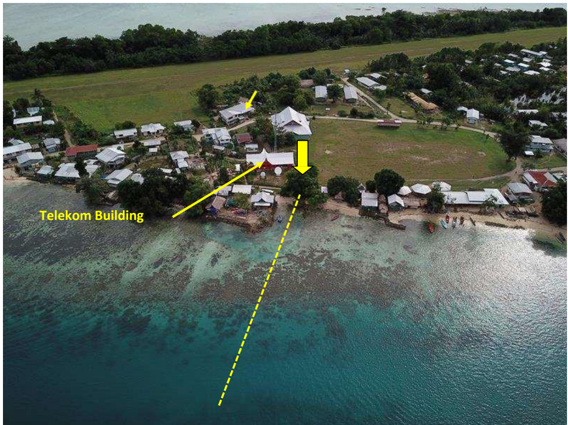
Figure 2-15 Aerial view of Taro landing point
