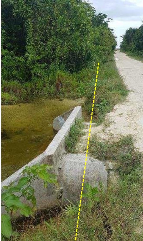
Figure 2-13 Crossing culverts over Langa-linga freshwater lagoon
