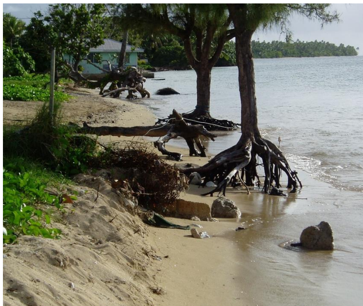
Figure 31 - Coastal erosion and undermining of front-line trees, Ha'apai
