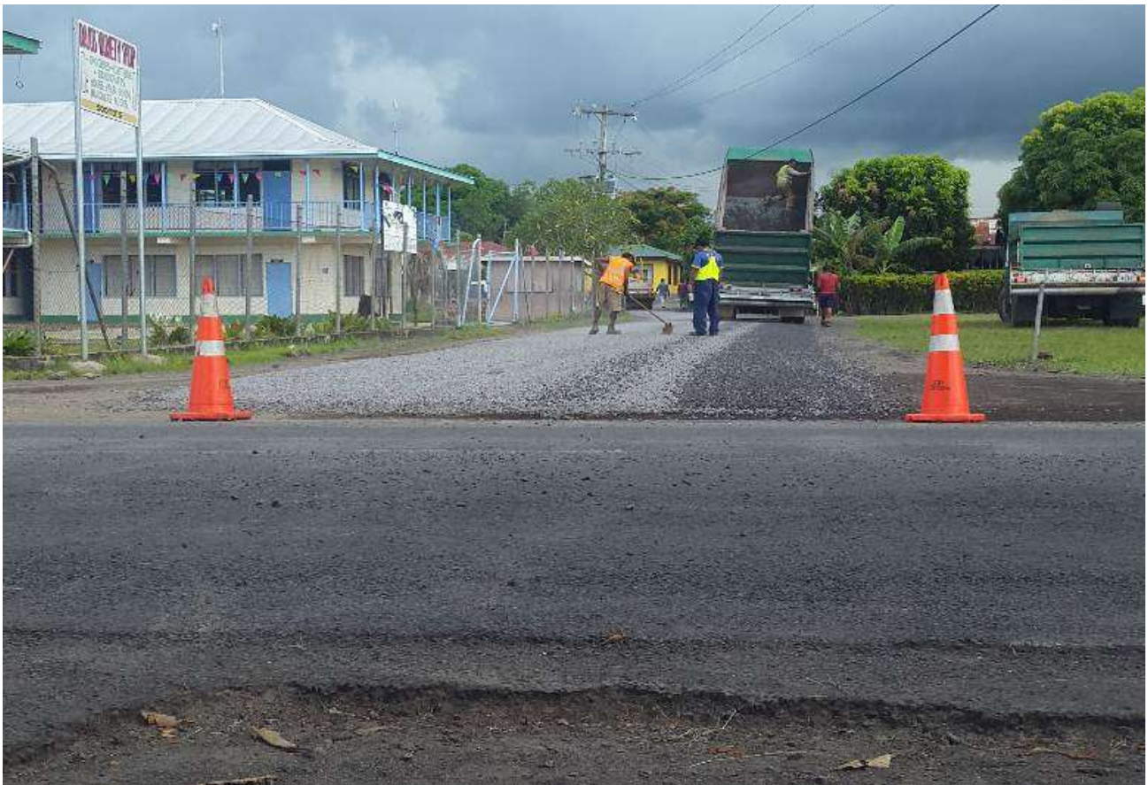
Nofaalii New Access Road completed in 2014 by LTA.
