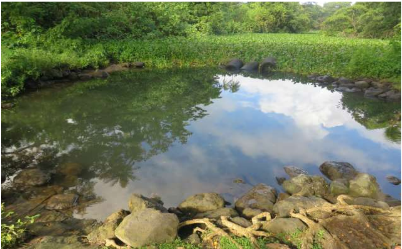
Invasive water lilies blocking the freshwater circulation within mangrove area and pushing culverts above water – need to remove lilies from pond
