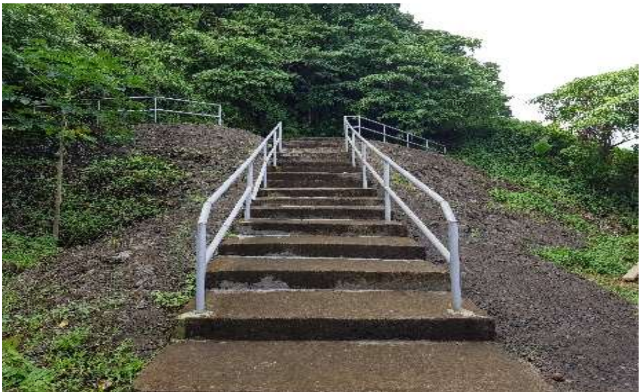
Staircase provided for the escape route behind houses on the coast at Saleapaga Village for tourist evacuation
