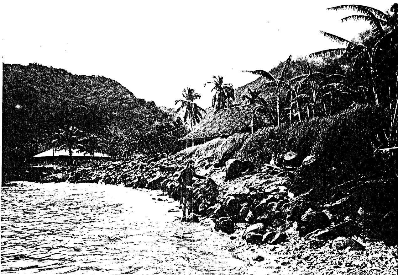
Fig. 9 - Afono Bay; boulder and cement seawall in front of school, incoming tide, looking from NW to SE.
