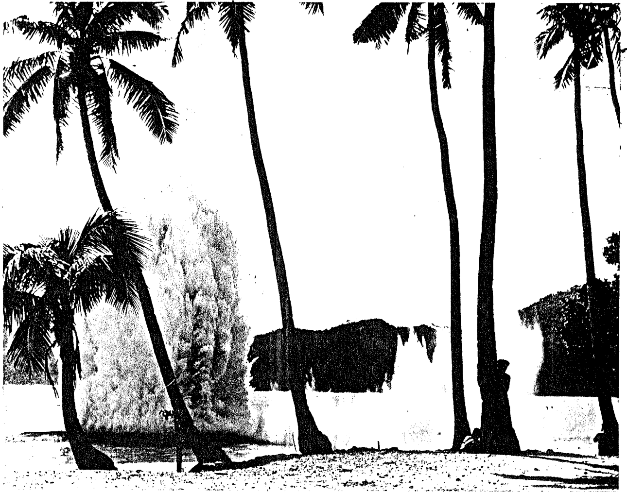
Fig. 20 - Aunuu Island; Explosive excavation N of Transect N, 16 March 1963, USS "Reclaimer" Project (courtesy of American Samoa Museum).
