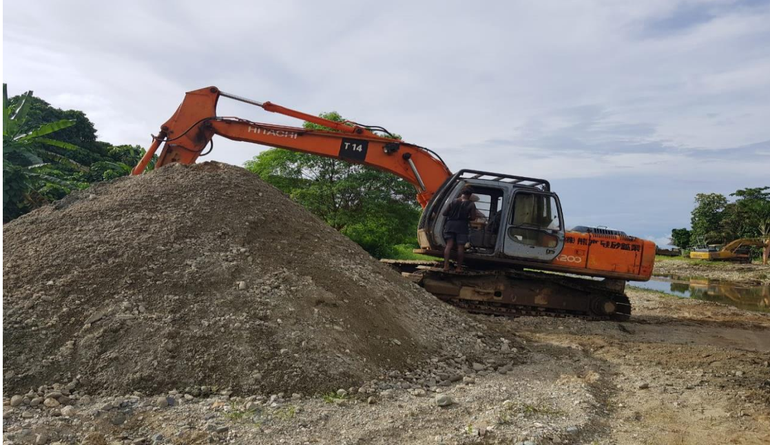
Figure 2: Gravel Extraction, Downstream Poha Bridge
