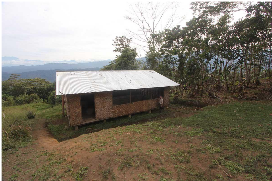
Plate 10. Naoro 2 – Elementary School building, 30 July 2014.
