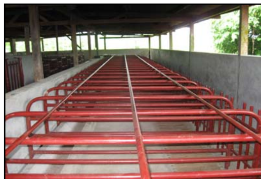
Interior dry stalls Building 2. Photo Credit: DLVS
