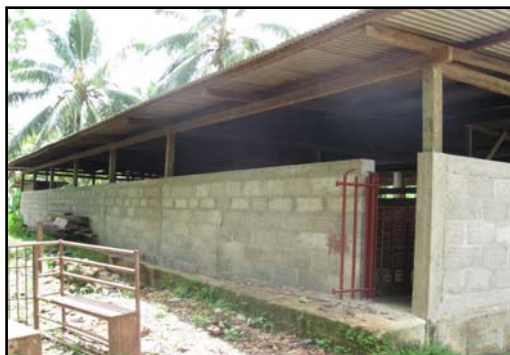
Side view of Building 1. Photo Credit: DLVS
