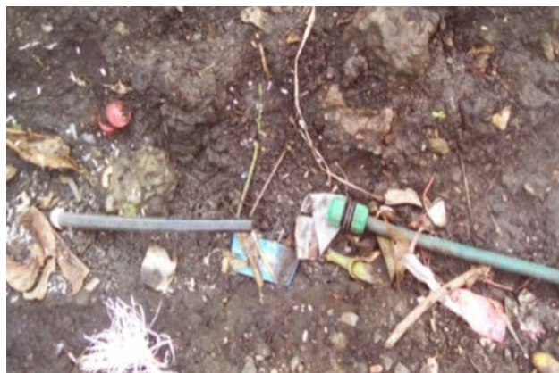
(Left) Illegal water usage (Right) Vandalized water pipe Photo © Susuki, W. and Newalli, J.
