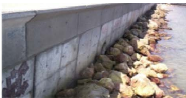
The seawall along Holy Parade Road, Koki Photo © Miria, G., 2012
